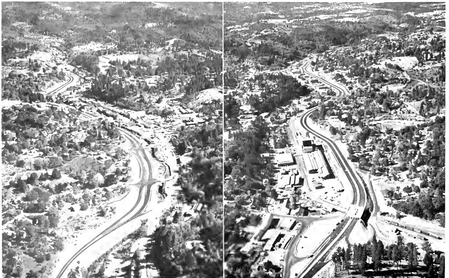
LEFT—Looking easterly at beginning of project. Old highway swings right across tracks and Hangtown Creek to follow Main Street. Spring Street (S.S.R. 49) crosses the expressway near center of picture. RIGHT—Looking westerly from near end of project. Washington Street Overhead in foreground. The structure spans relocated Washington Street, the Southern Pacific Railroad, and Emigrant Ravine. Placerville Fruit Growers pear packing plant, one of the world's largest, LEFT CENTER.
